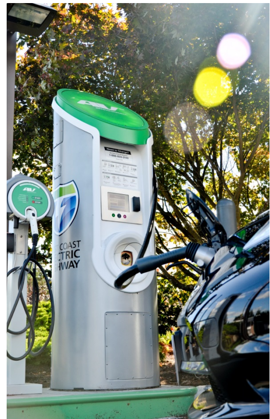
West Coast Electric Highway locations provide publicly-accessible Level 2 and DC fast charging.
